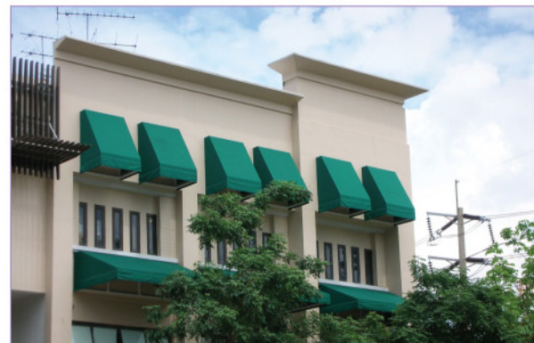
Building facade panel
