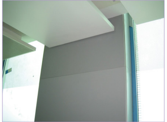
Wall cladding panels at Airport
