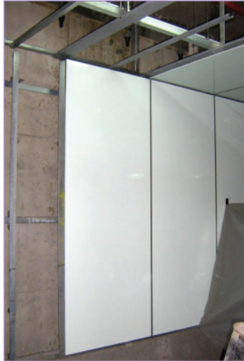
Wall cladding panels at MRT station
