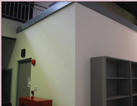
Heavy duty steel stud wall in workshop
