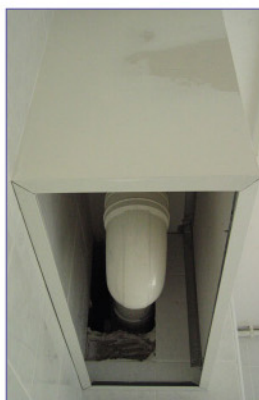
Casing for pipes & services
