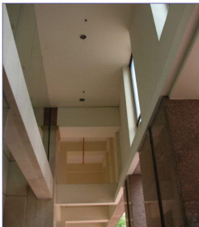
Semi-exposed concealed ceiling
