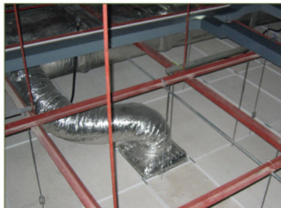
NuClad® grid ceiling system in biological clean room
