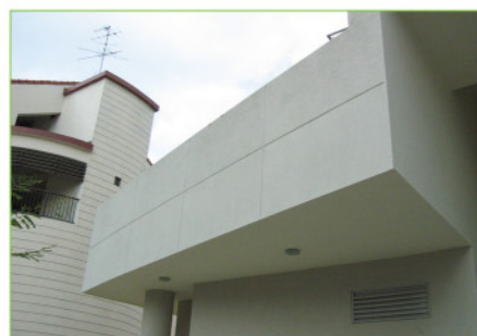
Building services enclosure with exterior paint finish
