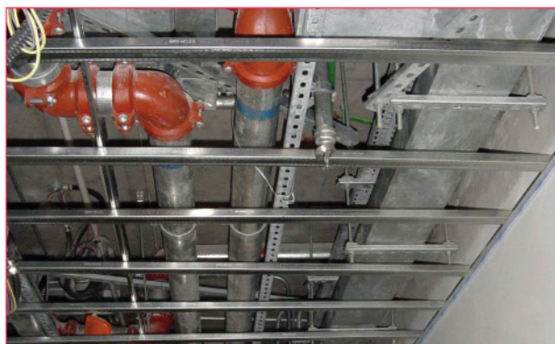
FP®-900/FirePro® fire rated building service ceiling enclosure
