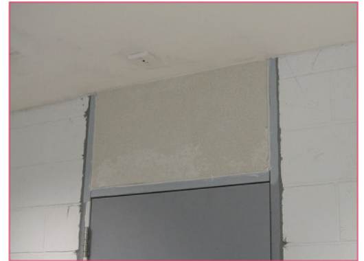
FP®-900 / FirePro® fire rated door overhead panel
