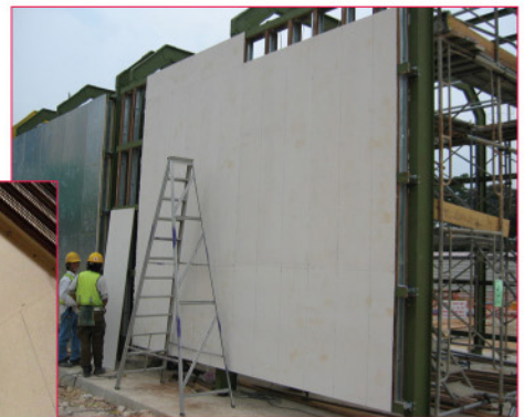
Fire rated industrial lining
