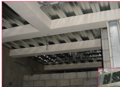
Beam encasement
